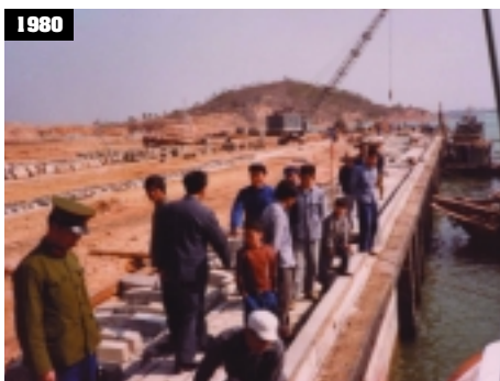
Building the quay wall at CIMC's first container factory in Shekou
