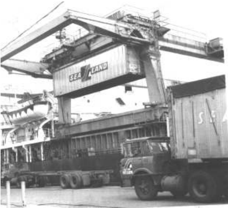
Sea-Land's early ship to shore container handling by ship-board container crane
