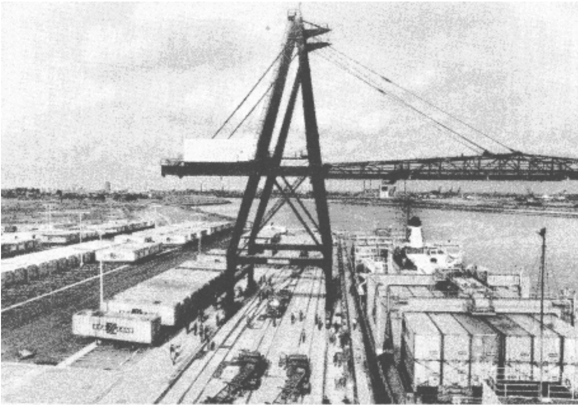
Sea-Land's Port Newark marshalling yard in about 1958, with one of the first cellular Container ships. The container ship had shipboard container gantry cranes. A dockside container crane was, however, available as well. The leading manufacturer of dockside container cranes was Pacific Coast Engineering Company (PACECO).
