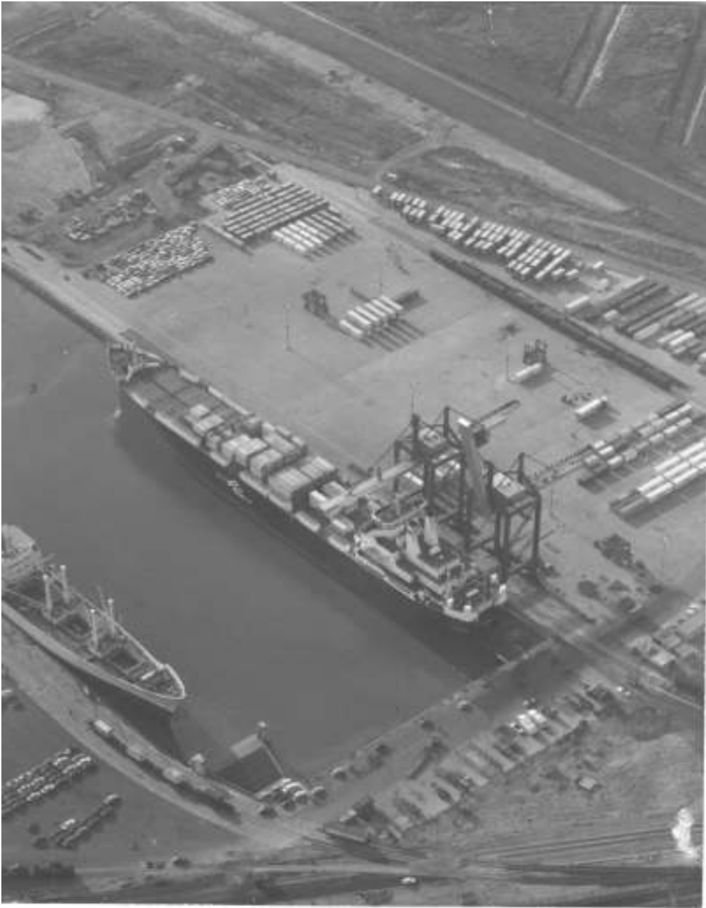
Bremerhaven's first container pier after completion
